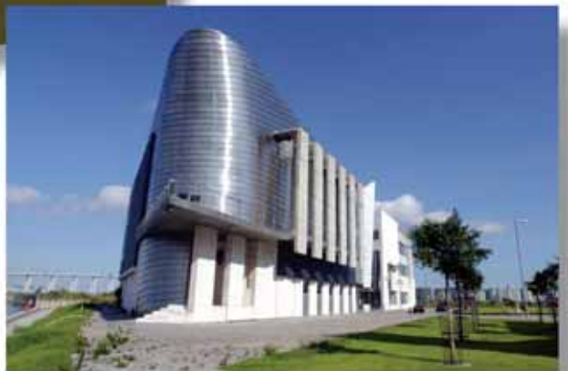
❖ The Court of Final Appeal and the Court of Second Instance Building
