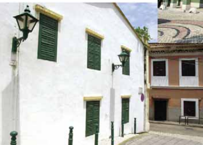
❖ Old buildings along Lilau area
