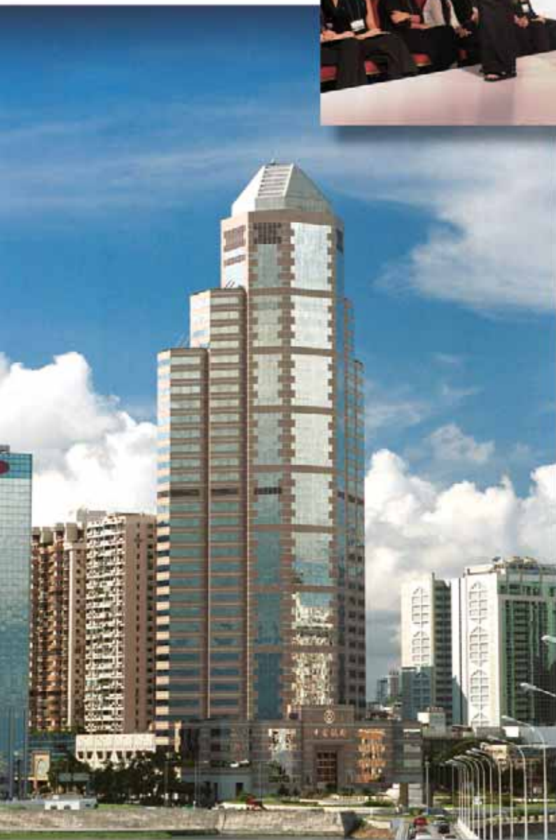
❖ The Bank of China Macao Branch Building
